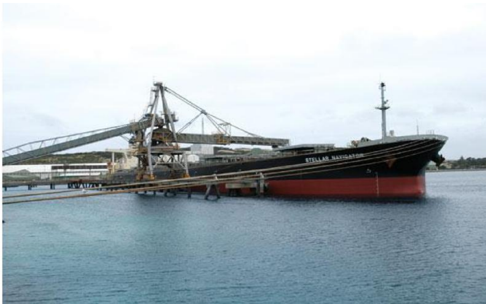
Figure 85. Iron ore loading at number 3 berth
